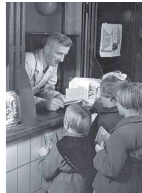
Savings counter at Zaandam post office, 1952
