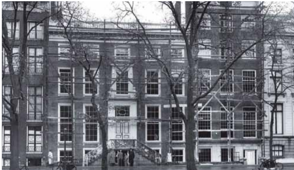
NMB head office during restoration, Herengracht, Amsterdam, 1937
